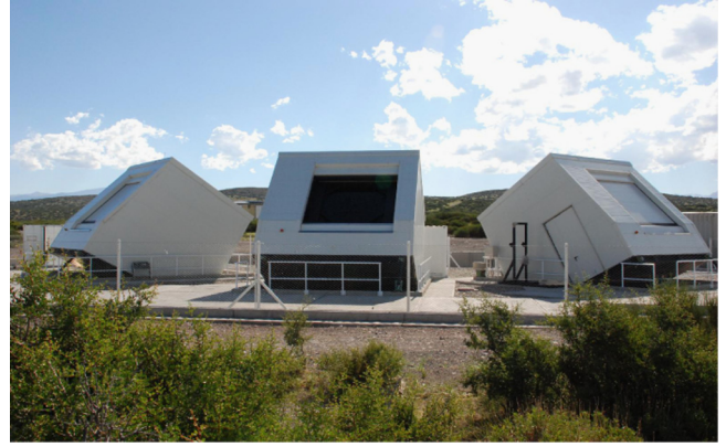
Fig. 50. Photo of the three HEAT telescopes in tilted mode. The container for DAQ, slow control, and calibration hardware is behind the enclosure of the second telescope.
