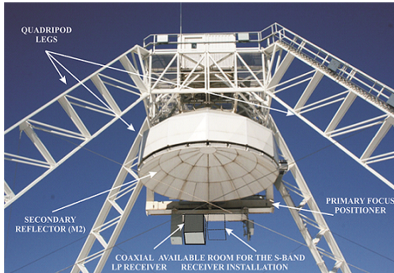
Figure 2. Detail of the sub-reflector and PFP of the Sardinia Radio Telescope. Two cubes depict the coaxial-feed LP band receiver that is already installed on the PFP and the available room for the S-band receiver.
