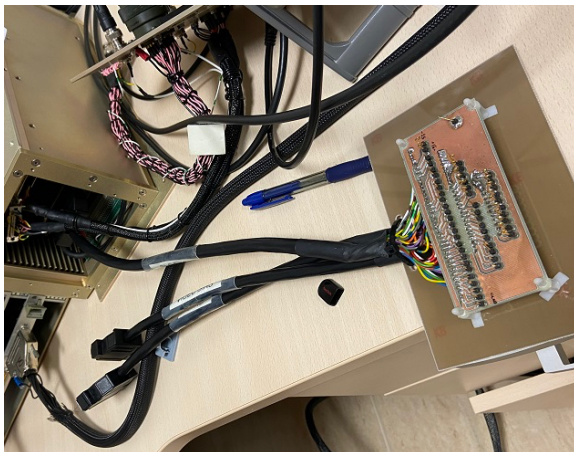
Figure 14 - ARC controller and Test Board
