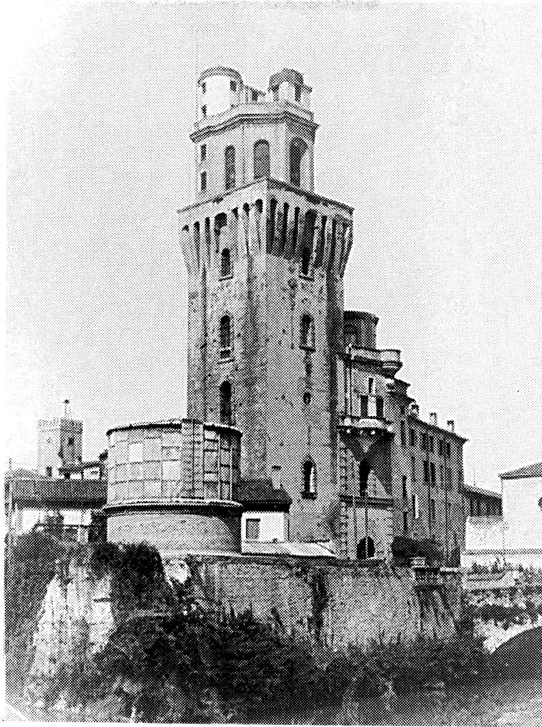
Figure 3. The high medieval tower transformed into the Padova Astronomical Observatory from 1767 to 1777. On the left is circular brick dome constructed in 1882 to house the Merz refractor (Photograph taken in 1929: Astronomical Observatory of Padova, Historical Archives).
