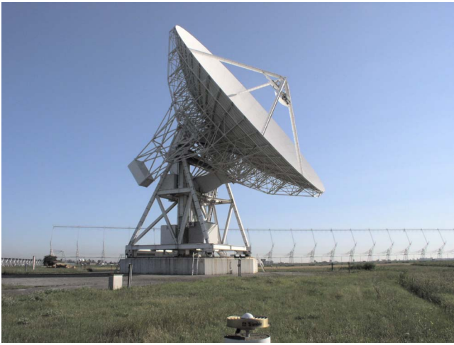
Fig. 1. 32-m AZ-EL VLBI radio telescope at Medicina; the VLBI telescope in Noto has the same design, structure, and dimensions
