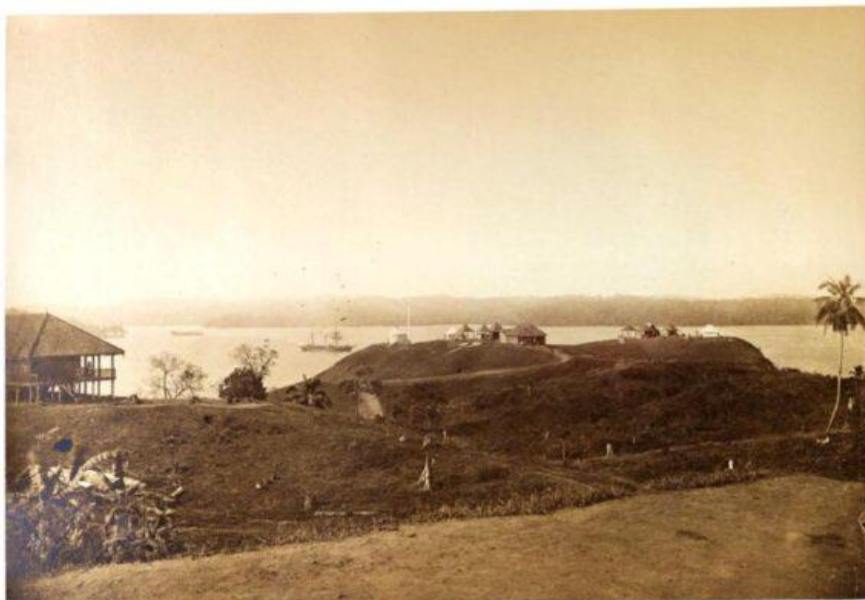
I. GENERAL VIEW OF THE OBSERVING STATIONS.
