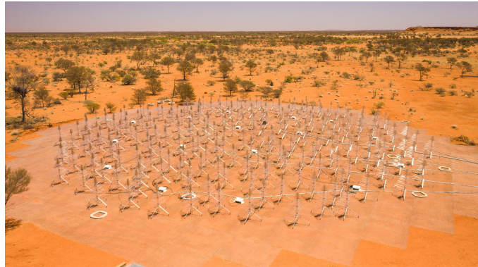
Fig. 1. An aerial view of the Aperture Array Verification System 2 (AAVS2), an SKA-Low prototype station deployed in 2020 at the Inyarrimanha Ilgari Bundara, the Murchison Radio-astronomy Observatory site.
