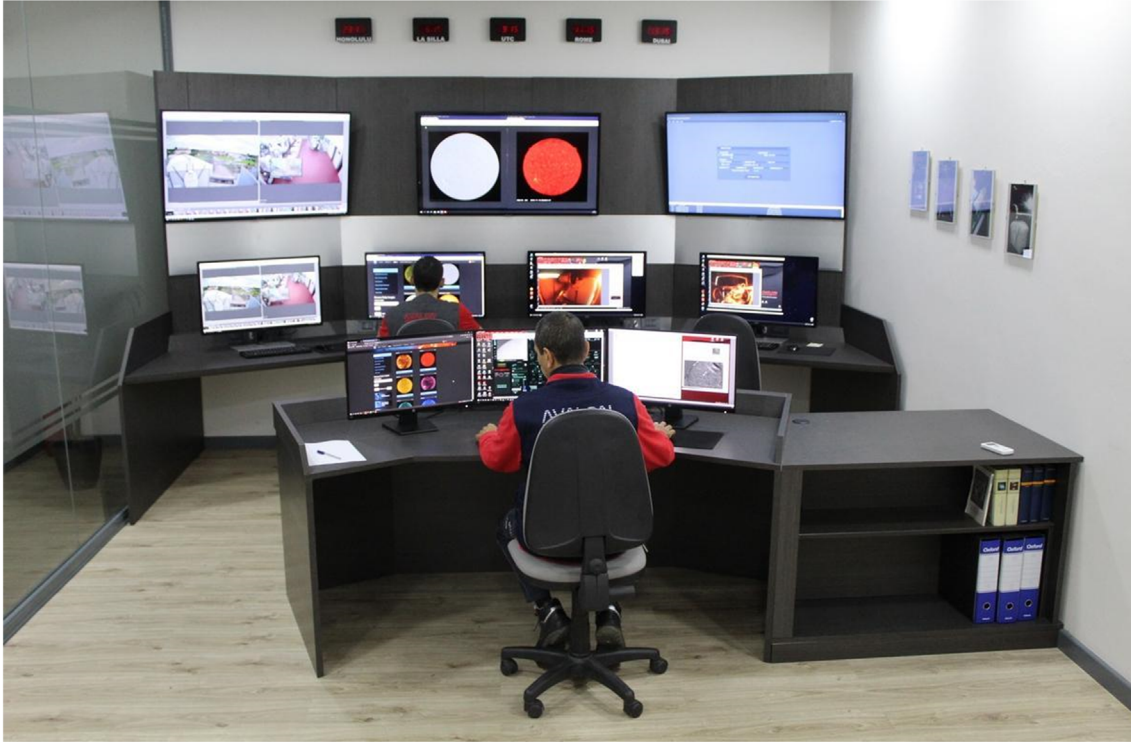
Fig. 2. The Avalon Instrument telescopes remote network control room.
