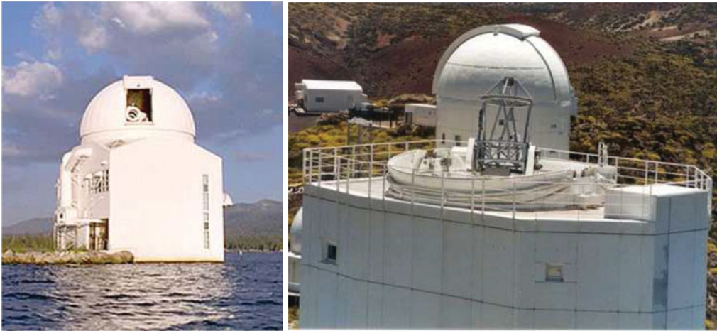
Figure 4. Left: the 1.6 m off-axis New Solar Telescope of the Big Bear Solar Observatory. The position on a pier within Big Bear Lake (CA) guarantees long periods of good to excellent seeing. NST has been operating since 2010. Right: the 1.5 m, on-axis German GREGOR telescope on Tenerife, inaugurated June 2012. The unique folding dome is visible, retracted on the floor of the building.
