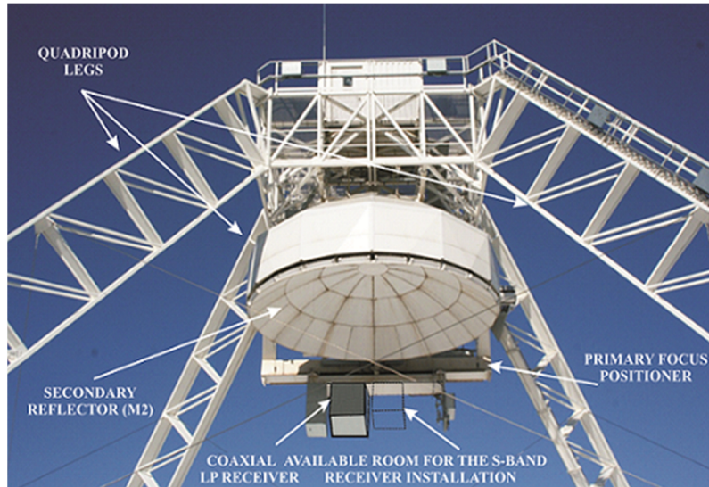
Figure 2. Detail of the sub-reflector and PFP of the Sardinia Radio Telescope. Two cubes depict the coaxial-feed LP band receiver that is already installed on the PFP and the available room for the S-band receiver.
