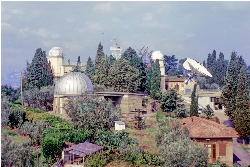
Fig. 17.5 The Arcetri Observatory seen from the Solar Tower in 1968. The image shows, from the right: the 10-m radiotelescope (installed in 1963); behind it, the 5-m radiotelescope (1962); next to the east (right) dome, the first Italian radiotelescope (1956); at the center, an antenna for satellite telemetry (Historical Archive, INAF-Arcetri Astrophysical Observatory).
