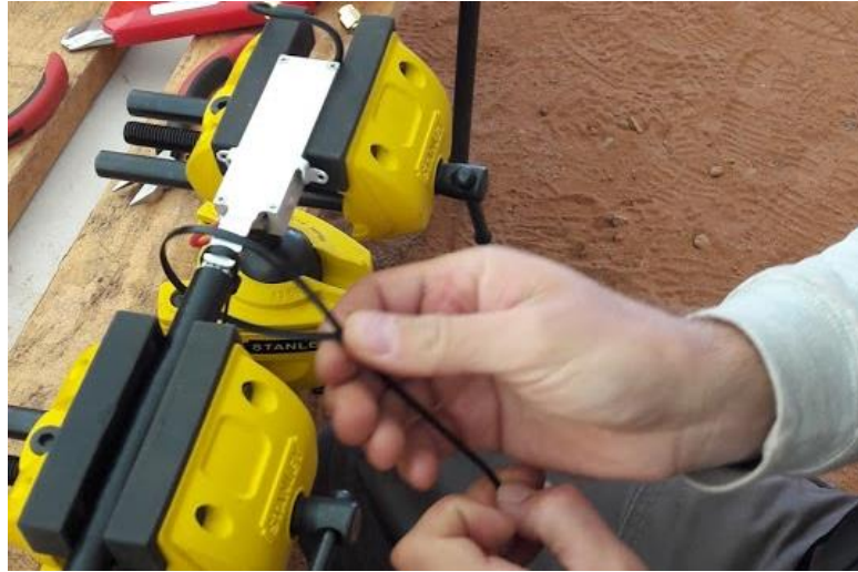
Figure 23: Cable ties tightening.
