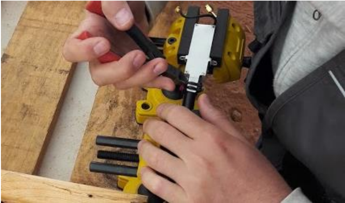
Figure 21: Cable ties cutting.
