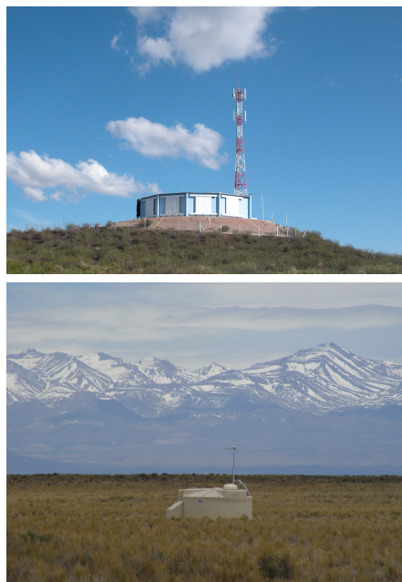
Figure 2: The fluorescence detector enclosure Los Leones (top); a surface detector station (bottom).
