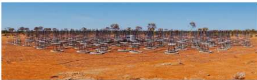
Figure. 1 Photograph of the prototype station in Western Australia
