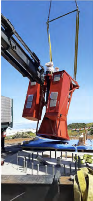
Figure 11. Installation of the telescope basement at the ASTRI site (left) and assembly of the M1 dish (right).
