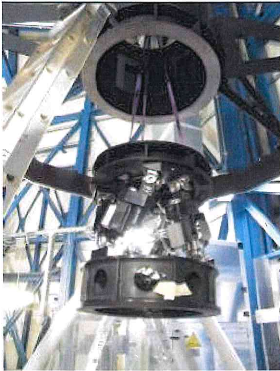
Fig. 6 – A phase of the installation of the hexapod in the telescope.
