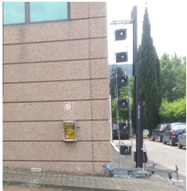
Fig. 8. Deployment of the ANC system at the corner of a building.
