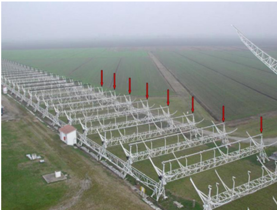
Fig. 1: The eight parabolic reflectors making up the BIRALES-Rx array within the Northern Cross, in Medicina, near Bologna, Italy
