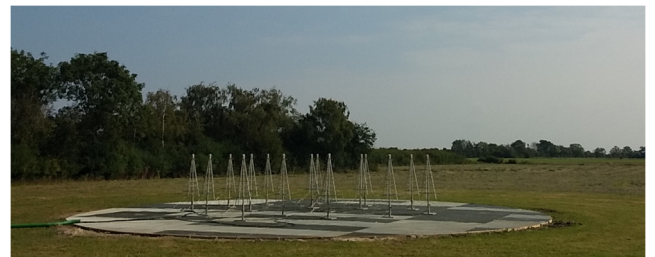
Figure 3. Picture of the AAVS0 array. The array was installed over a platform covered with a metallic mesh.
