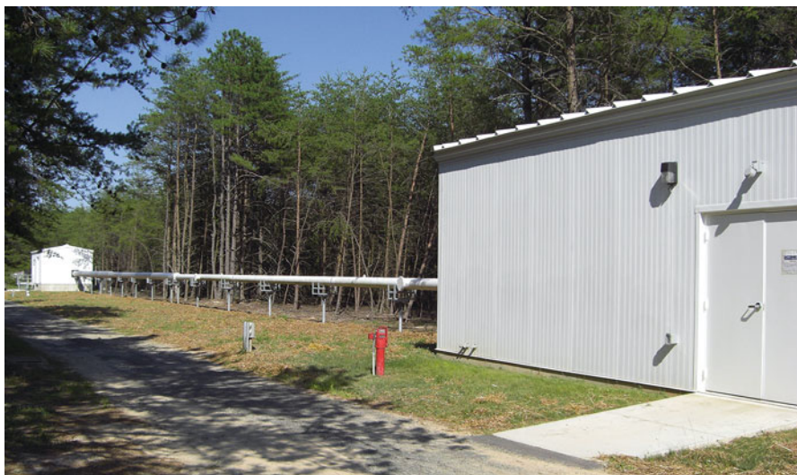
Fig. 16 Image of the GSFC 100-m X-ray beamline showing the X-ray source and instrument buildings. (Credit: NASA GSFC)
